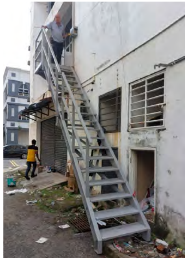
Fire Escape Staircase for PDK Damansara Damai
